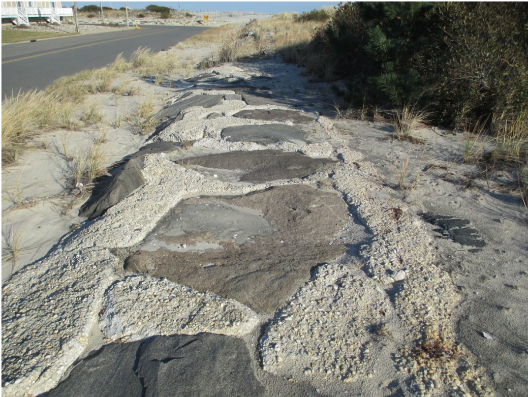
Figure 7: Typical seawall construction from Philadelphia Ave to Wilmington Ave.
