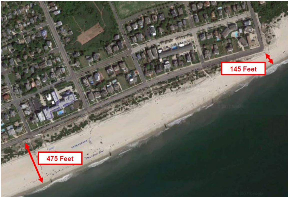
Figure 19: Distance from the seawall to the ocean at Beach and Wilmington Avenue Area.
